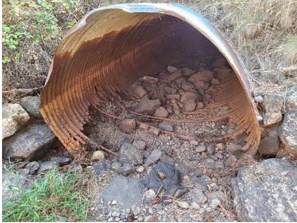
Figure 28: Lincoln Rd culvert deterioration
