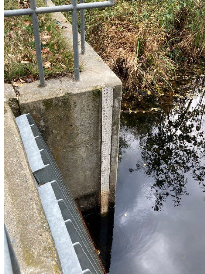
Figure 4: Outlet channel gage is beginning to deteriorate at water level.
