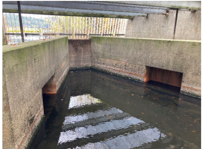
Figure 2: Flood gates need to be repainted. Surrounding concrete shows some pitting.
