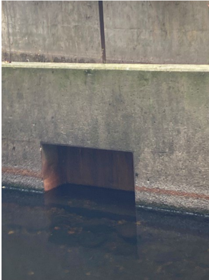
Figure 3: Northern gate is leaking slightly.
