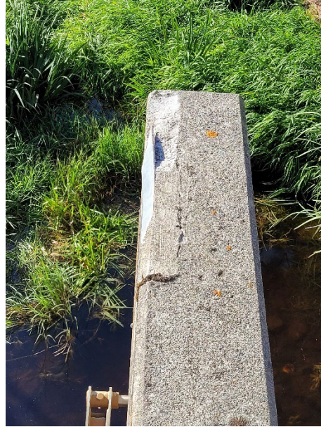
Figure 14: Concrete spalling at the top of the roll gate and corner of abutment.
