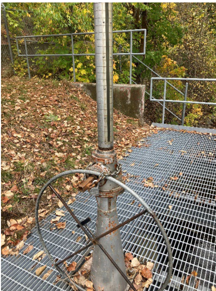
Figure 1: Gate wheel showing signs of rust.
