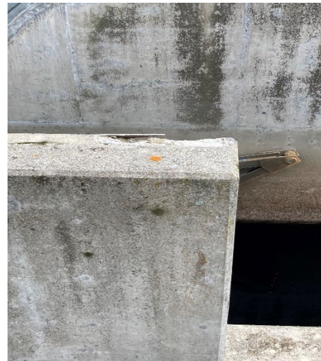
Figure 16: Spalling viewed from otherside
