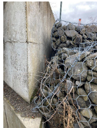
Figure 20: Gabion baskets at southwest and northwest corner of Starr Road Bridge are pulling away from the bridge.
