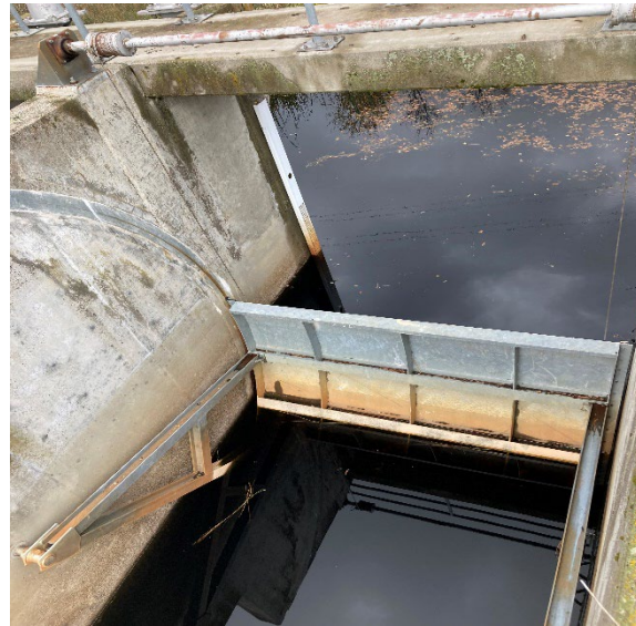
Figure 18: Radial gate closed during facilities inspection, viewed from above.
