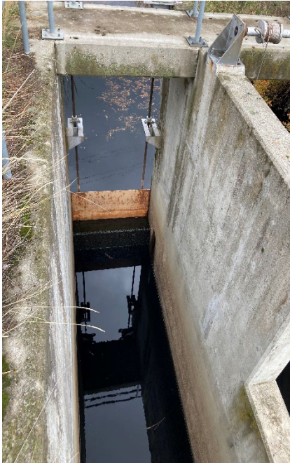
Figure 17: Weir gate closed during inspection.
