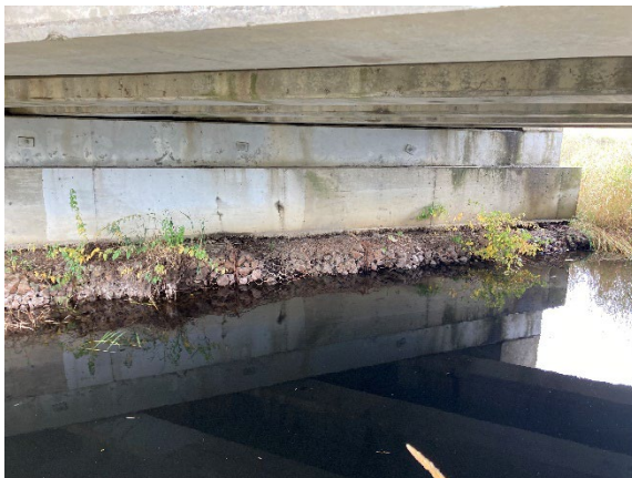
Figure 19: Gabion baskets beneath the bridge deck are separating from the bridge and deteriorating.
