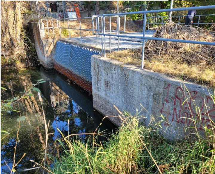
Figure 6: Concrete spalling and pitting along with graffiti on upstream side of the outlet structure.
