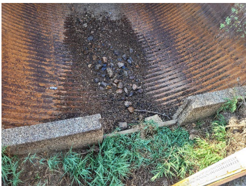
Figure 25: No weir boards are present.
