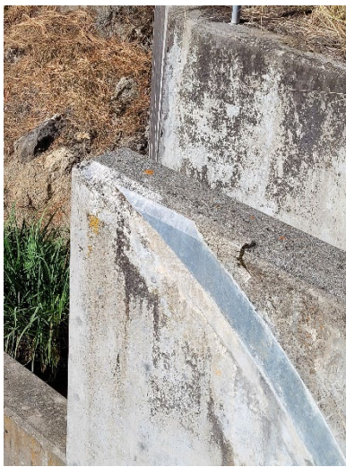
Figure 15: Spalling on roll gate
