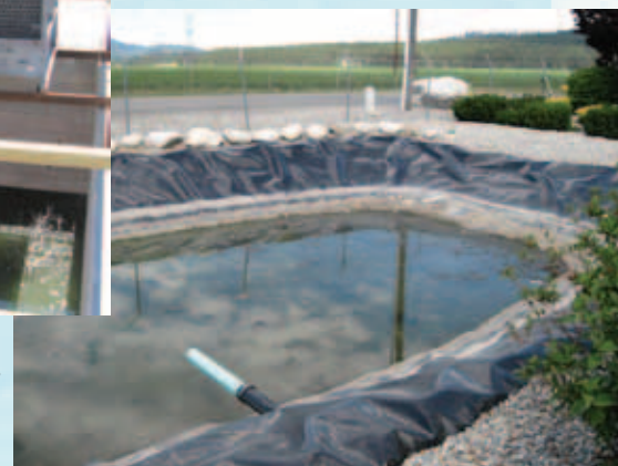
Passive wastewater evaporation pond
