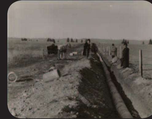
Laying irrigation pipes, 1908
