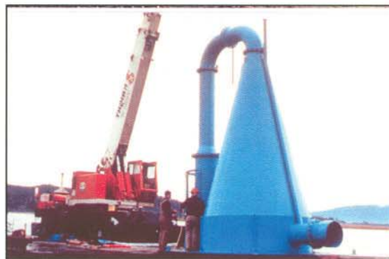
Aerator Construction 1992 – Installation of Speece Cone
